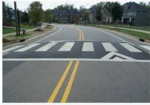
Figure 28. Example Crosswalk on Road Hump.
