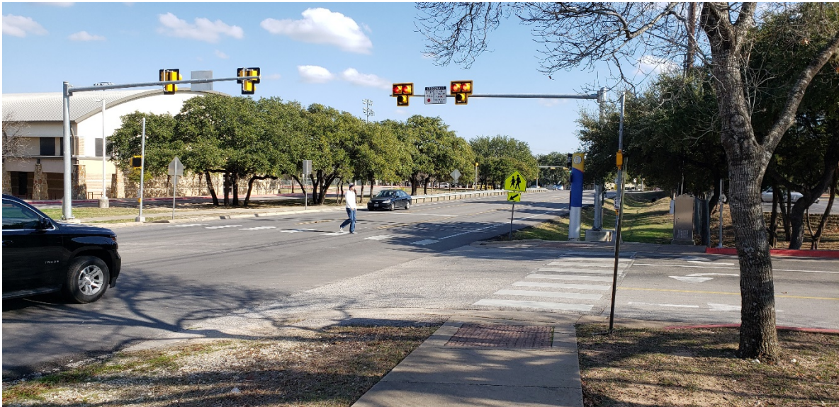
Figure 21. Pedestrian Hybrid Beacon (PHB)
