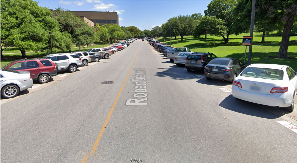
Exhibit 7: Robert Dedman Drive Before Improvements
